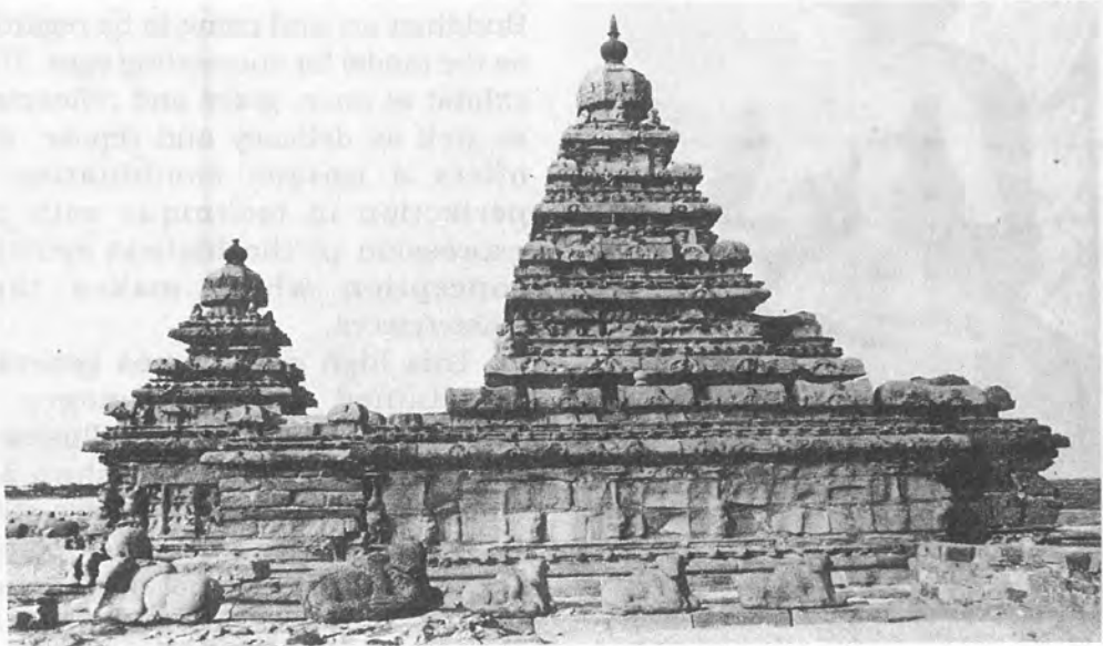
Fig. 19.7 Shore Temple at Mamallapuram
