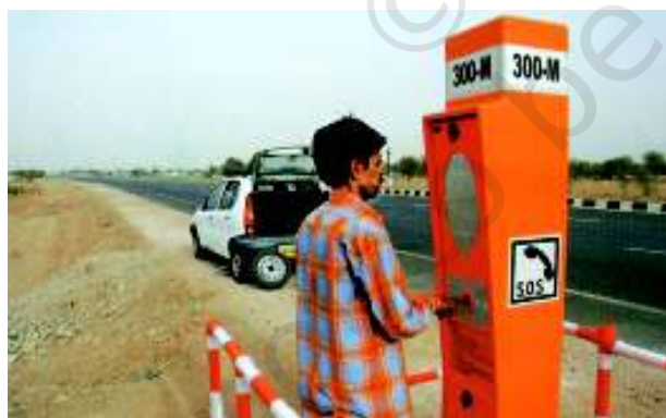
Fig.7.10 : Emergency call box on NH-8
