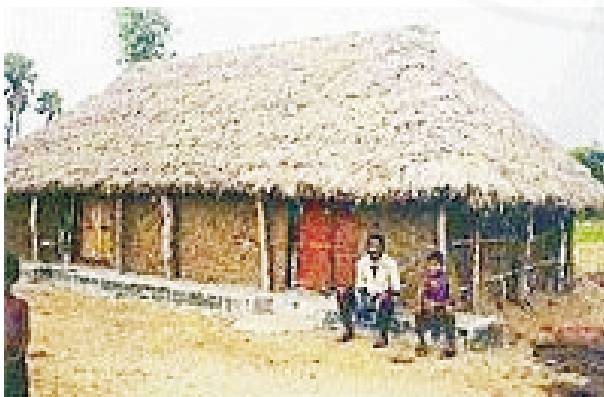
Fig 2.3.7 A shelter with special feature to withstand cyclones and floods. Traditional homes can be improved by building in disaster resistant features. Such homes could withstand cyclones with moderate speeds.
