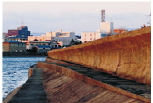
Fig 2.2.5 Tsunami walls in populated coastal areas of Japan
