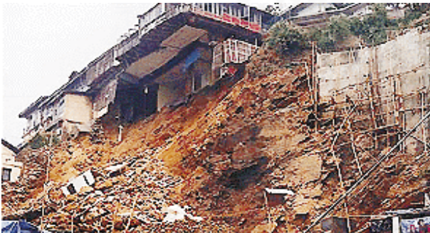
Fig 2.6.1 Landslide in hilly terrain of India
