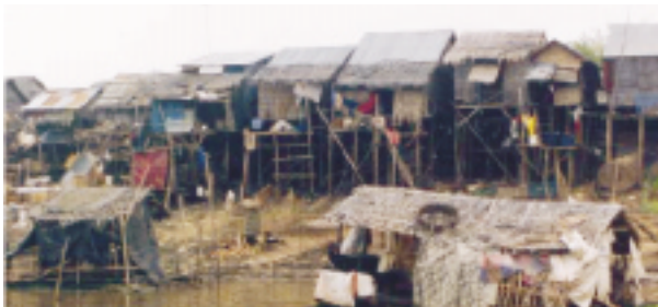
Fig 2.4.2 Houses constructed on stilts in slum areas
