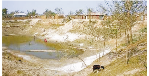
Fig 2.4.3 Khash Dhalai Flood Shelter.
