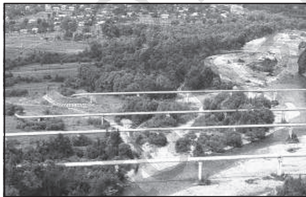
Fig. 8.17: Pipelines transporting natural gas in Ukraine
