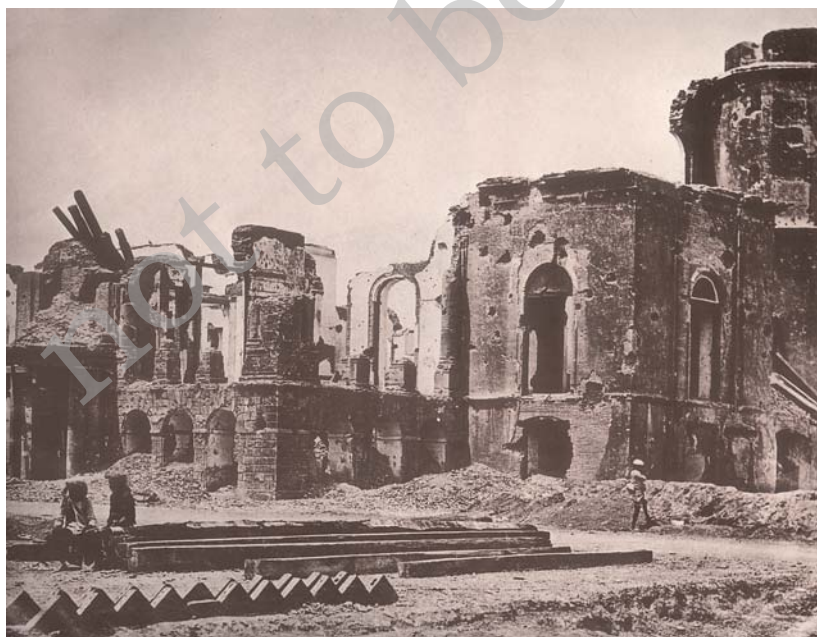
Fig. 12 – Ruins of the Residency in Lucknow
