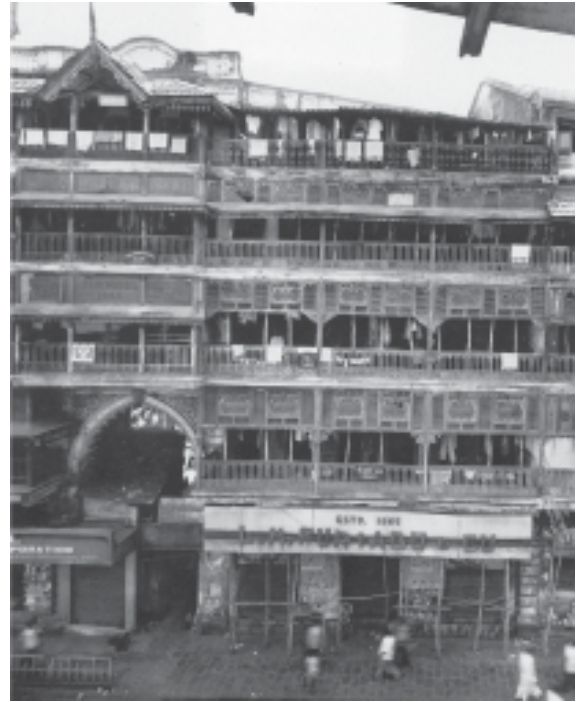
Fig. 21 – Chawl on Kalbadevi Road built in the early twentieth century. What do you notice about the organisation of space in this building?
