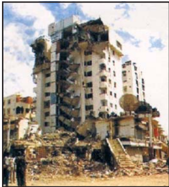
Fig. 3.3a: Destruction caused by an Earthquake in Gujarat
