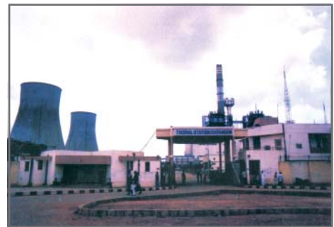
Fig 3.12: A view of a Thermal Power Station
