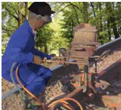
Figure 3.11 Thermit process for joining railway tracks
