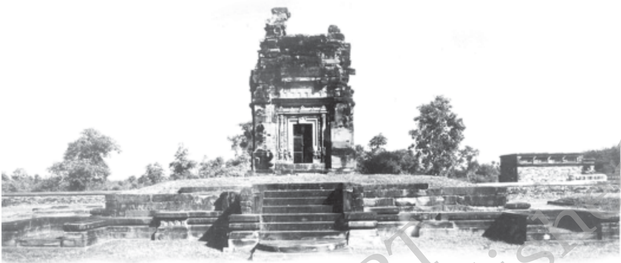
Fig. 4.25 A temple in Deogarh (Uttar Pradesh), c. fifth century CE
